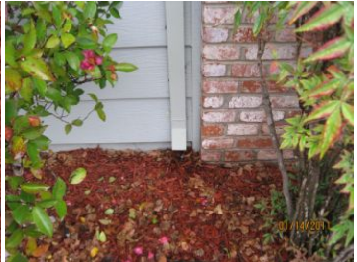
divert water away from foundation
