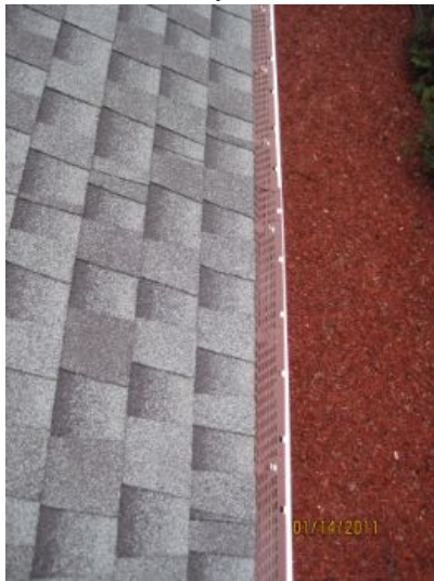
gutter guards in place
