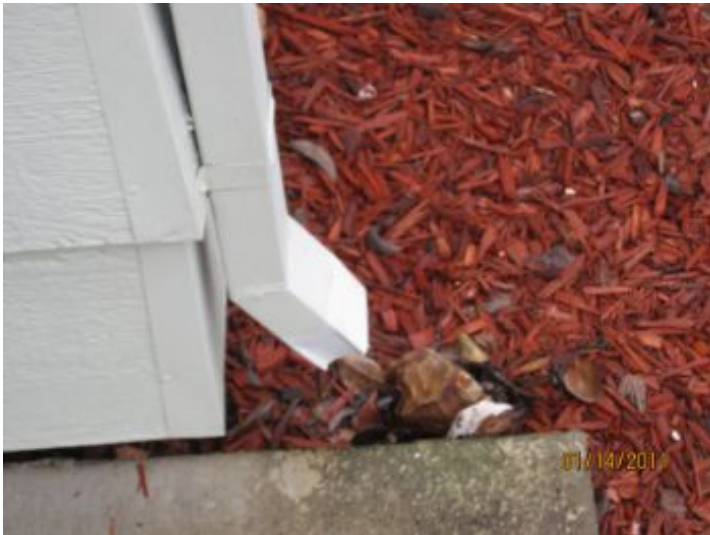
divert water away from foundation
