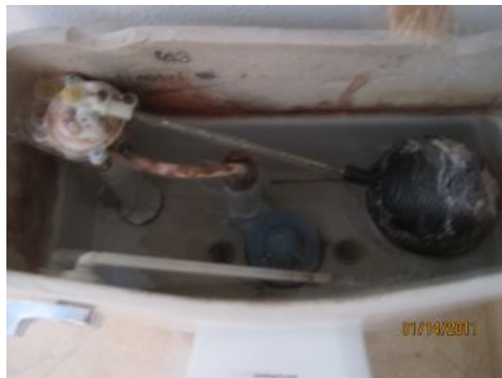
older toilet in guest bath
